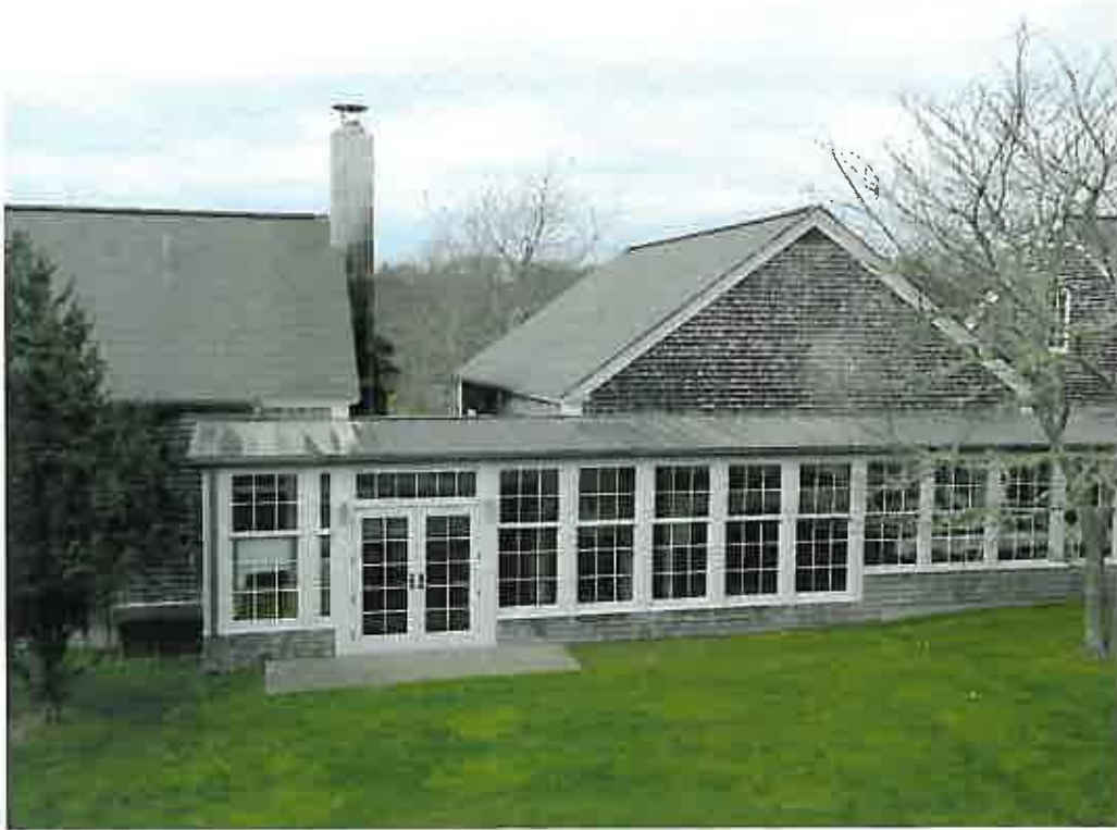
OVERVIEW OF SOME OF THE ROOFING AT THE CHILMARK SCHOOL
