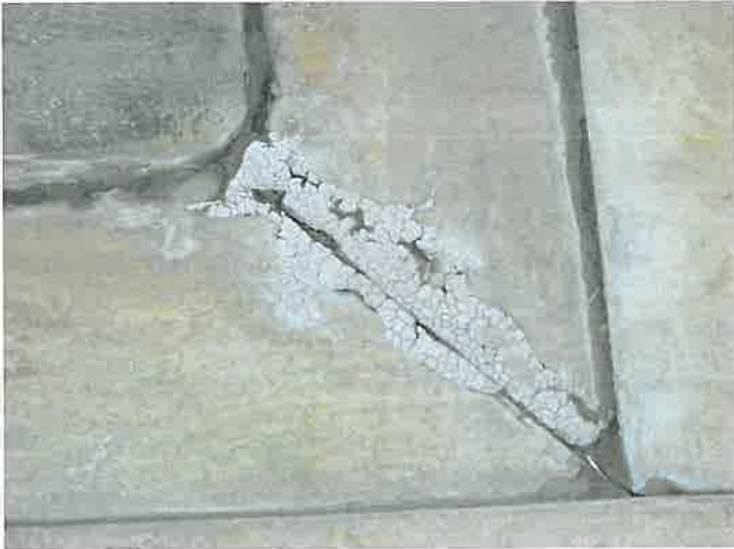
EVIDENCE OF SEALANTS USED AT THE LOW SLOPED LEAD COATED COPPER ROOF
