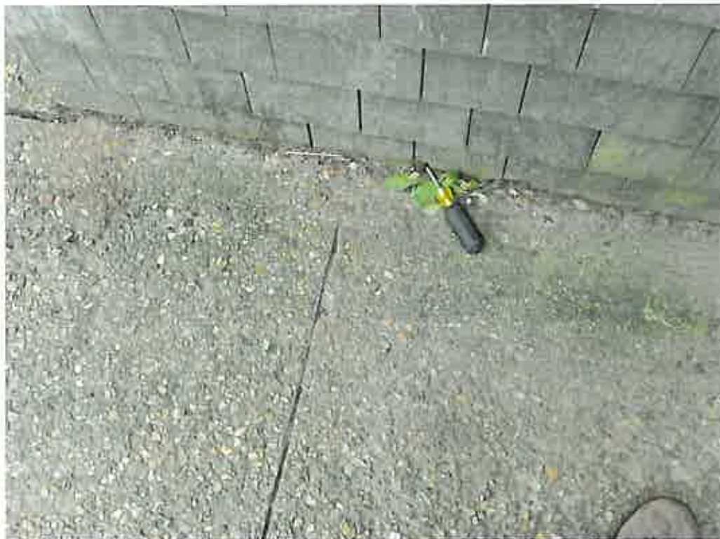
DETERIORATED SIDING IN CONTACT WITH A CONCRETE WALKWAY
