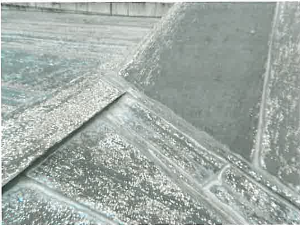
MORE SEALANT USE AT THE LCC LOW-SLOPED ROOF
